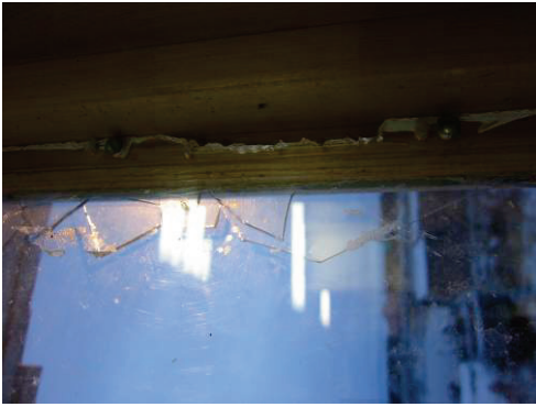
Damaged Plexiglass Window Replacement
