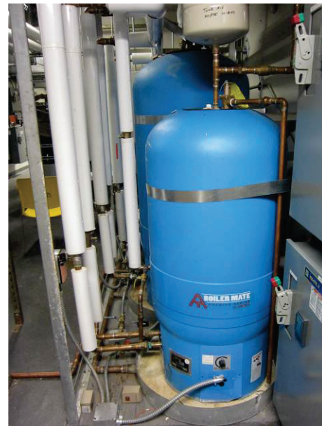
Amtrol BoilerMate Water Heaters
