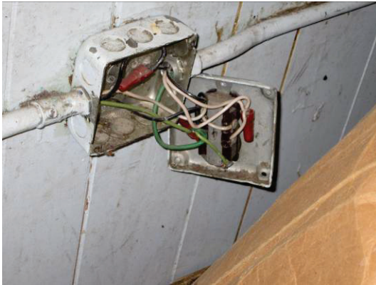
Exposed Wiring
