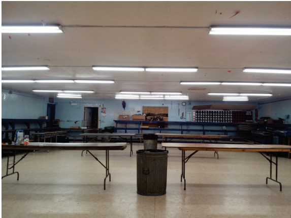
T8 Lighting Upgrade
